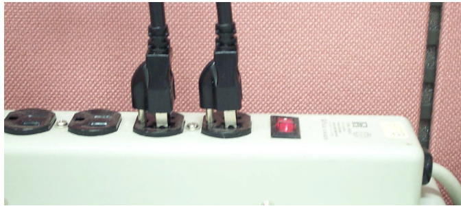
Figure 3.6: Power cord plugs should have same orientation in the socket/ 插座上电源线方向相同 / 插座上的電源線方向應相同
